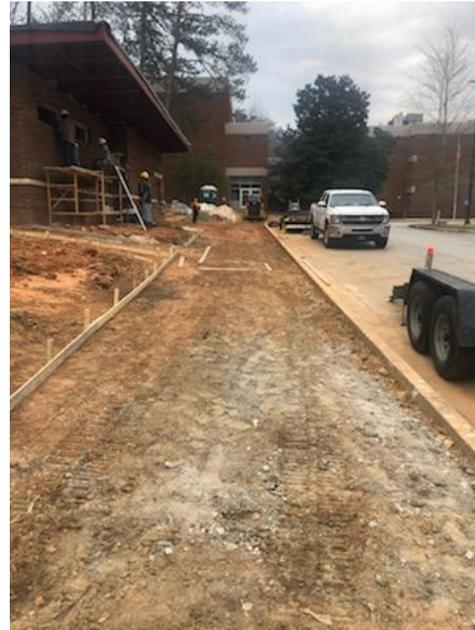
*Figure 2 S. Atl – Grading for Sidewalks*
