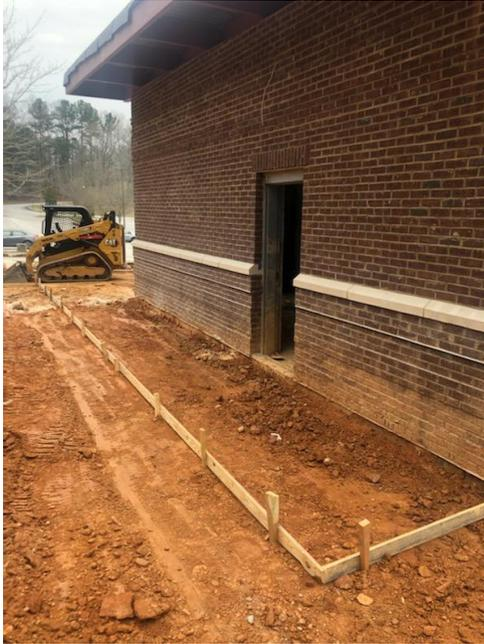
*Figure 1 S. Atl –Grading for Sidewalks*
